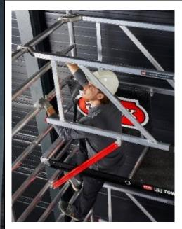
Access the working platform internally through the scaffold by climbing through the hatch deck using the rungs of the end frames as a ladder.
