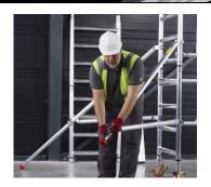
Ensure stabiliser clamps are secured tightly on the frame.
